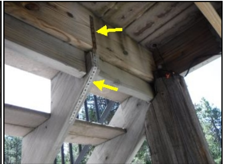
Improper attachment of stair stringers.
