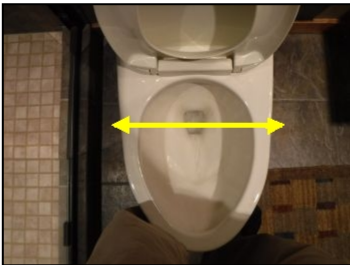
Upper level, hall bathroom toilet was loose. Mounts needed to be addressed.
