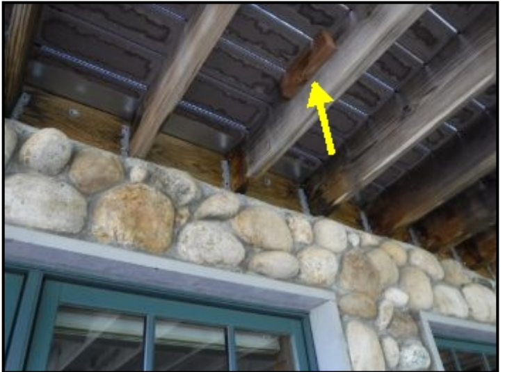
Deck boards had shrinkage.
