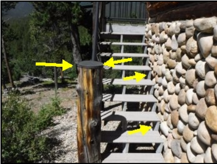
Safety Hazard. Stair stringers have failed/cracked through. Stair treads are loose and may fail at any time.
