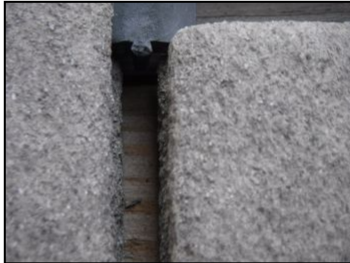
Decking was deteriorated.
