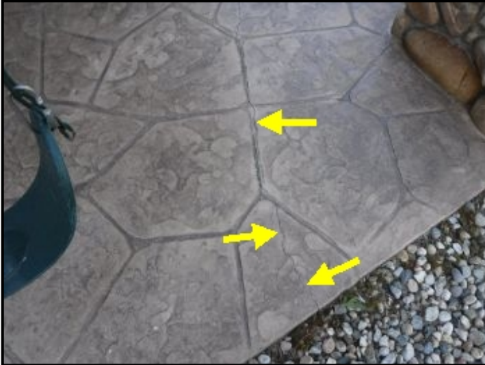
Back/west patio: Settlement cracks noted.
