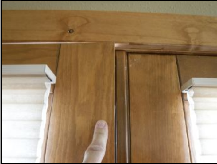
Lower level living room door was binding in the frame.
