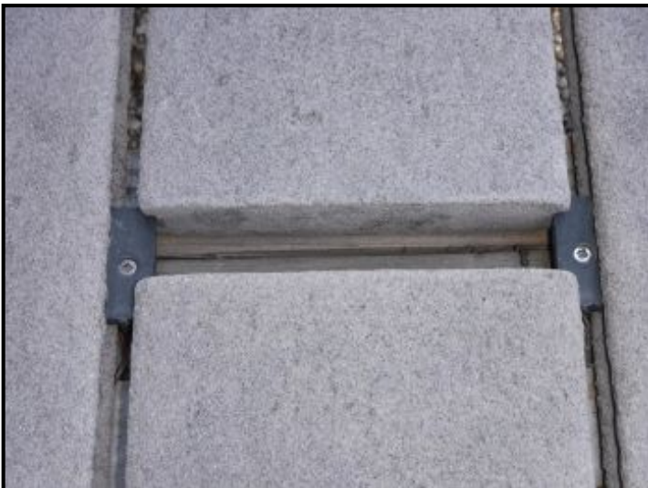
The composite deck boards were significantly deteriorated. Consider replacement of the deck surface.
