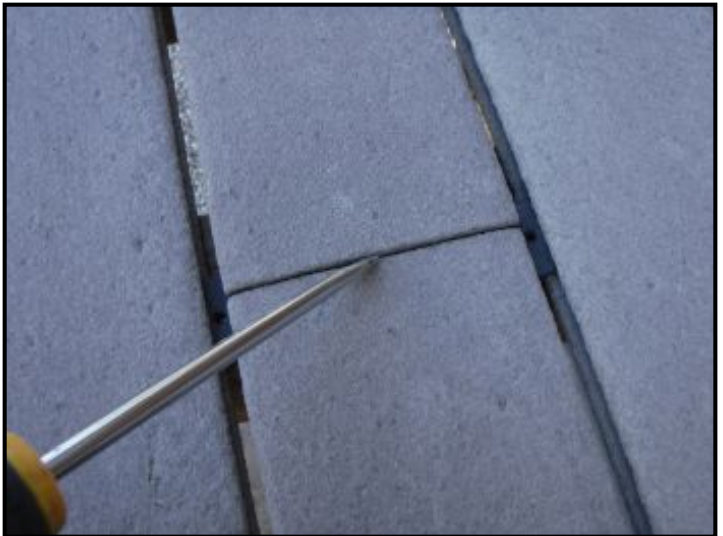
Some deck boards were not secure.
