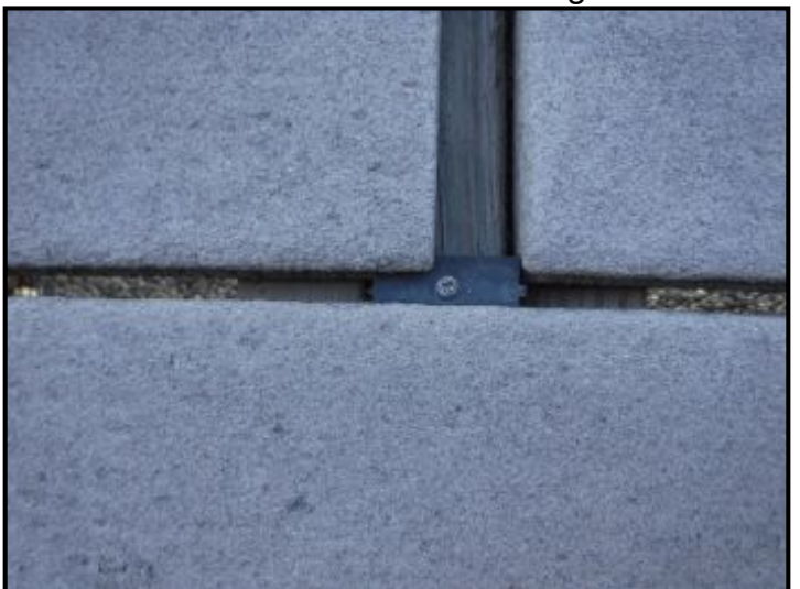
Deck boards had shrinkage.
