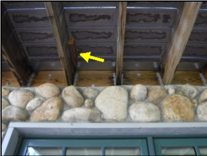
2" x 4" 's used to support deck boards that apparently have shrunk with time / reduced in length over time.
