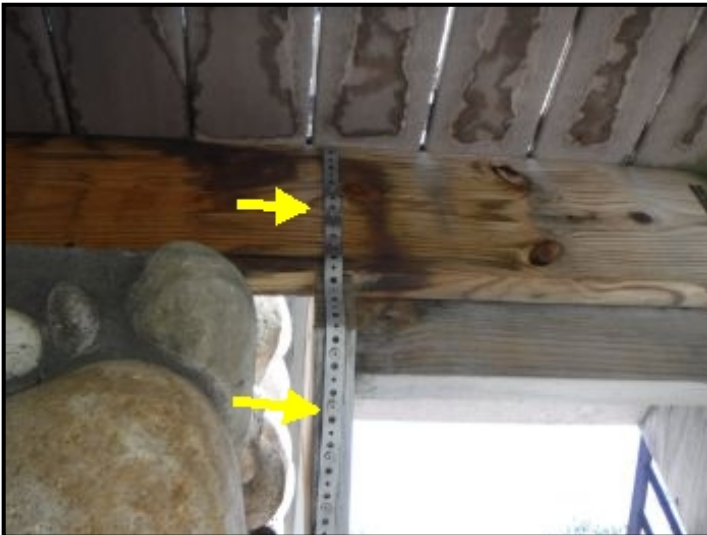
Improper attachment of stair stringers.
