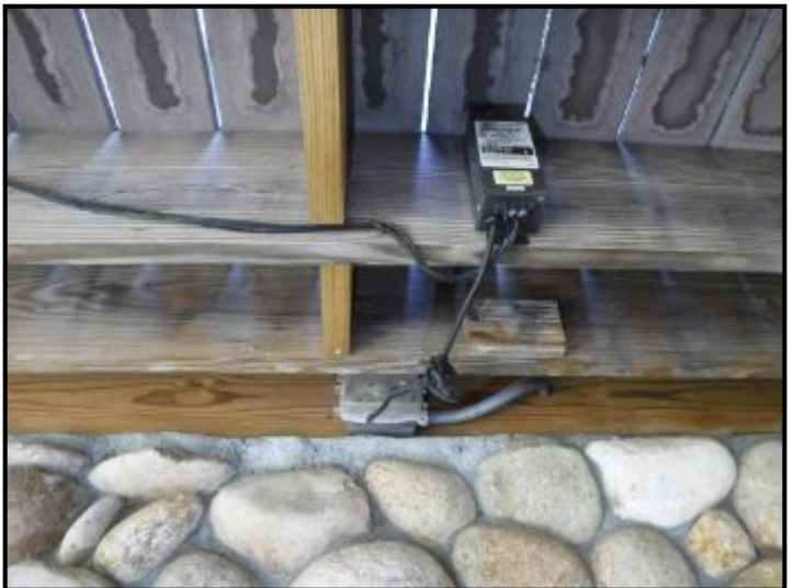
Exterior wires should be enclosed in conduit.
