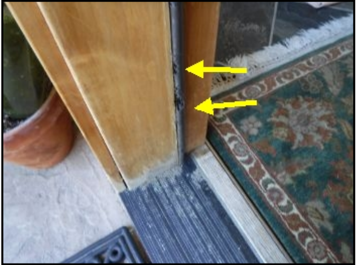
Main entry door, weather strip was damaged.
