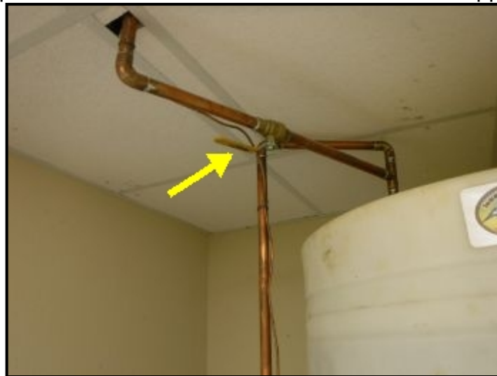
Water shutoff valve location.
