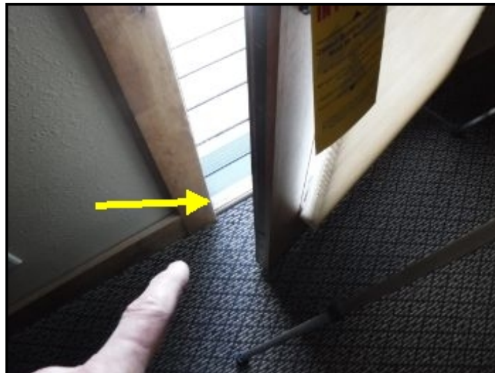
Office, upper level, door to deck was binding at the threshold.
