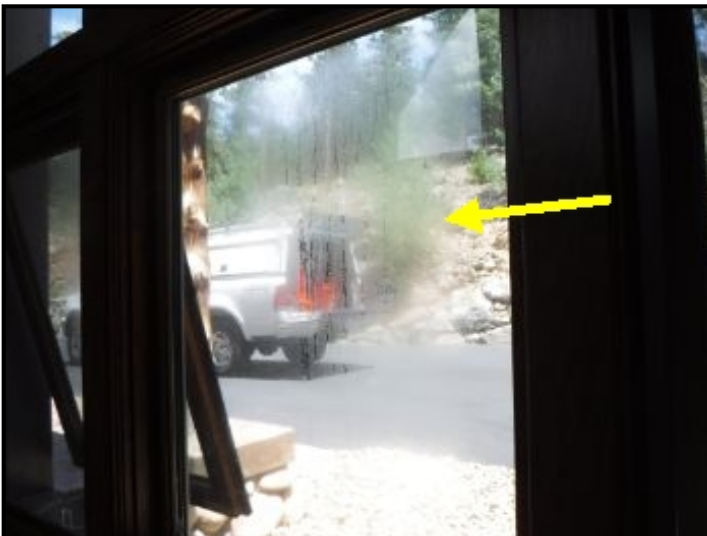
Condensation present in some double-paned windows, indicating a broken gas seal.
