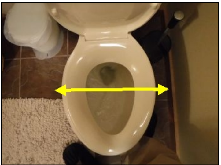
Lower level, south bathroom, toilet was loose. Mounts needed to be addressed.
